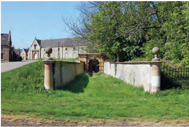
The tunnel entrance near the riding school. Photo Peter Turner. Reproduced from Geograph under creative commons licence
